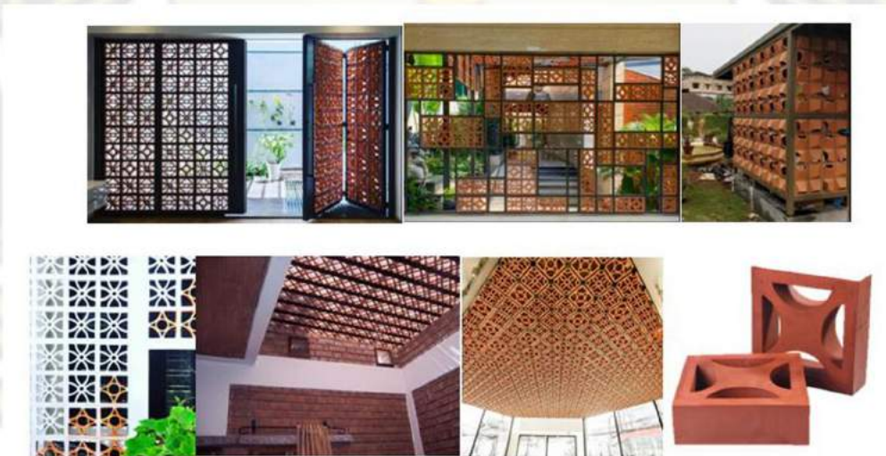
Fig: Application of Terracotta jali in building
